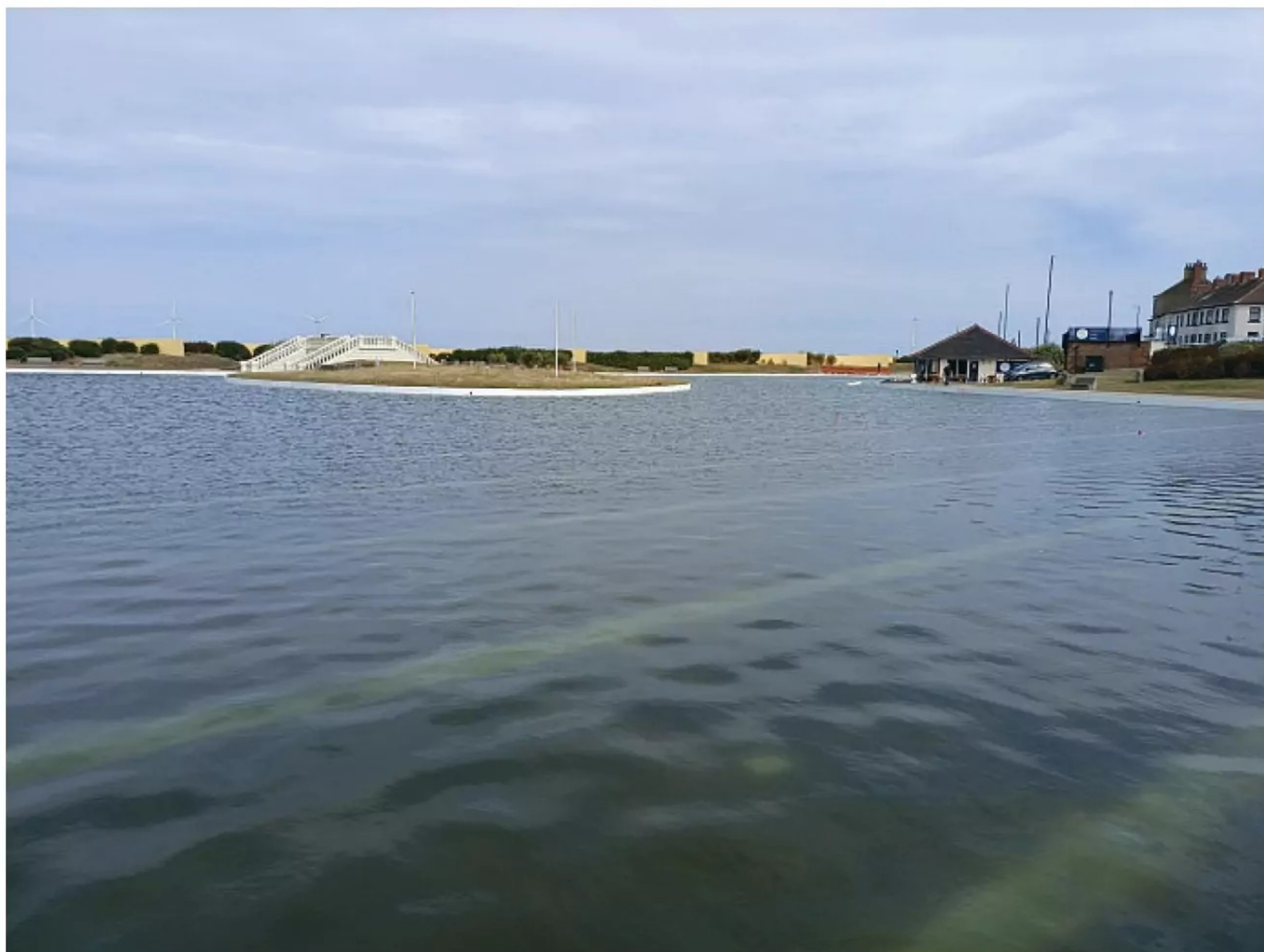
Congratulations to Redcar Model Boat Club, whose members can finally enjoy sailing again on the newly repaired and filled Coatham Lake!
