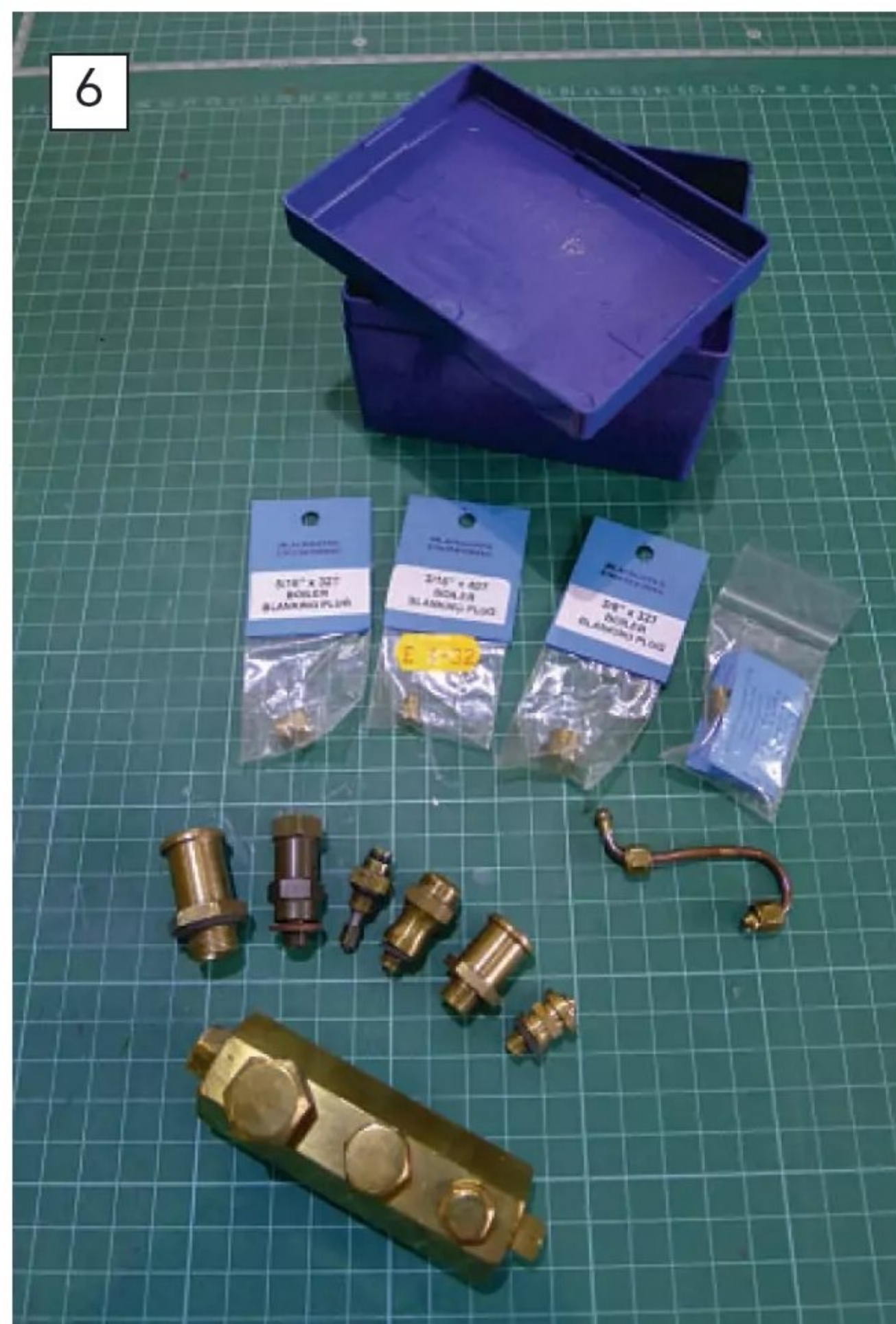
Richard's first little plastic box contains frequently required bits and pieces, such as safety valves and plugs. The safety valves are just emergency stand by units, because if a valve was changed out for a steam test the boiler would need retesting again if it was replaced. Richard is happy to let them go on long term loan if necessary!
