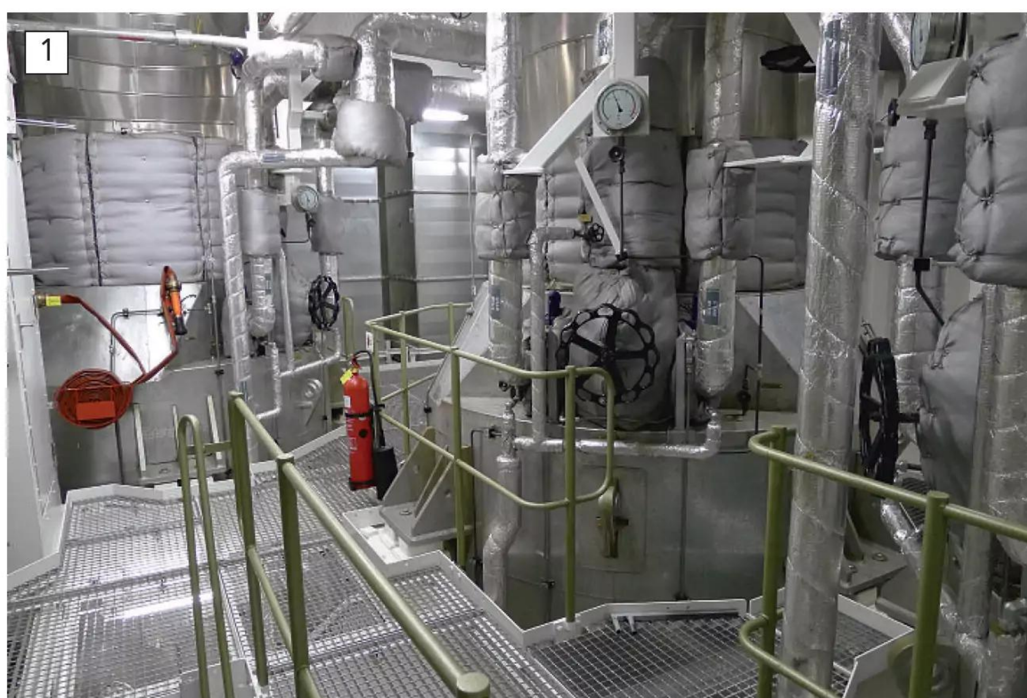
Standard marine practice is to insulate all surfaces of a boiler with thick rockwool lagging, clad in aluminum sheeting, as well as all steam pipework, valves and fittings. Wasted heat is directly related to wasted fuel.
