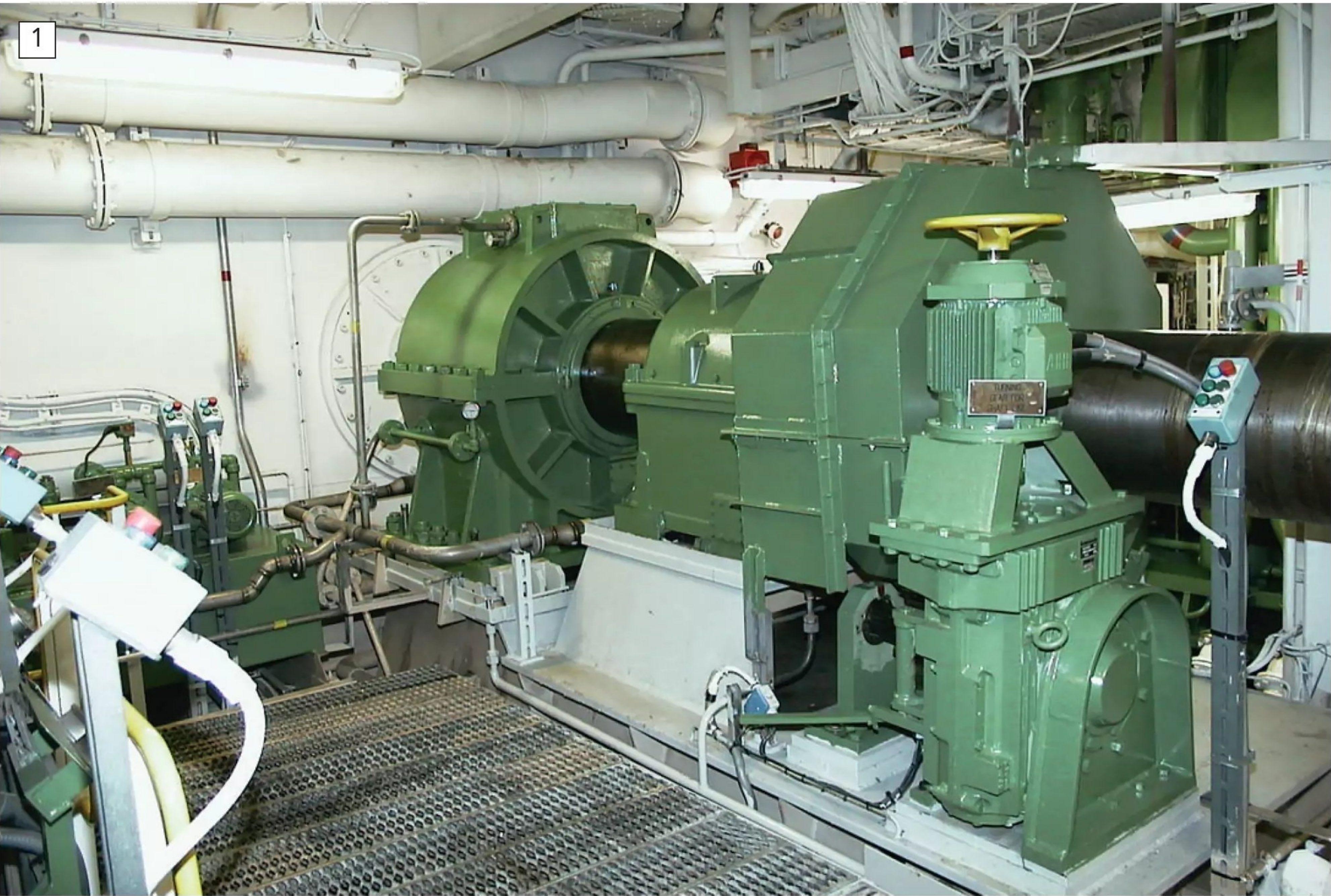
A modern main propulsion shaft showing clearly, from right to left, the shaft turning gear, an intermediate bearing and the main thrust block.
