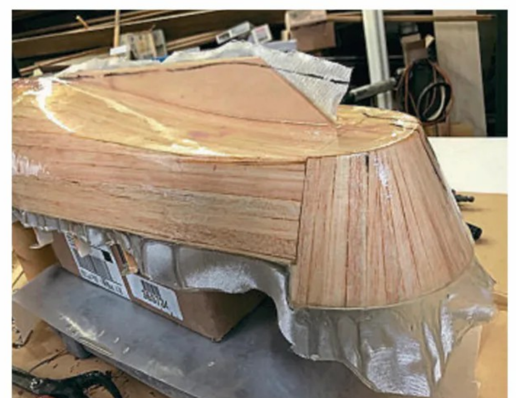
Fibreglass cloth should be cut so that it fits easily in place, particularly when compound curves are involved.
