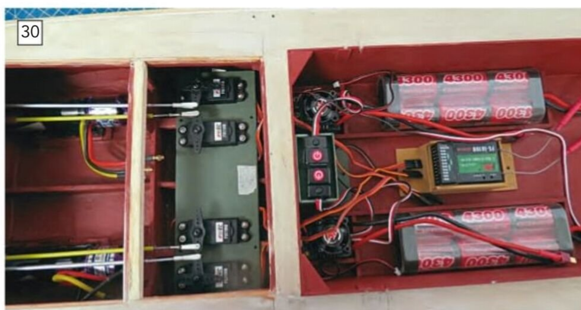
All the electrical control and power systems finally in position.
