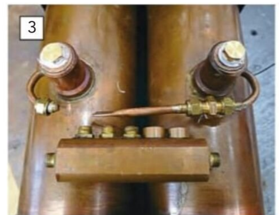
Because the plant has a single engine, the two boilers are connected together with a manifold on the steam outlet lines to supply steam to the engine, as well as a number of other users of steam.
