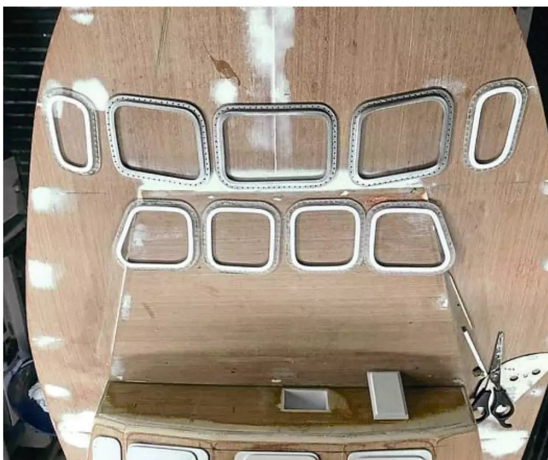
Work in progress on the window frames.
