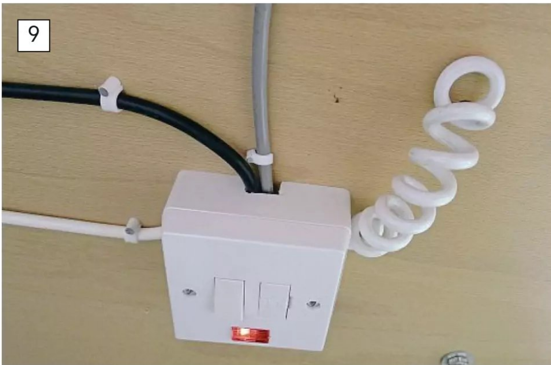
A fused supply feeds the lathe, the milling machine and the grinding wheel, and sits neatly below the workbench.
