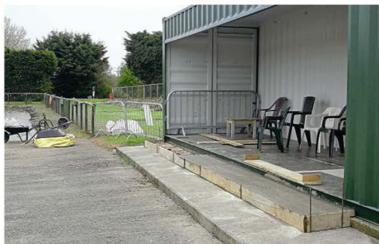
The new shelter with the extra step under construction
