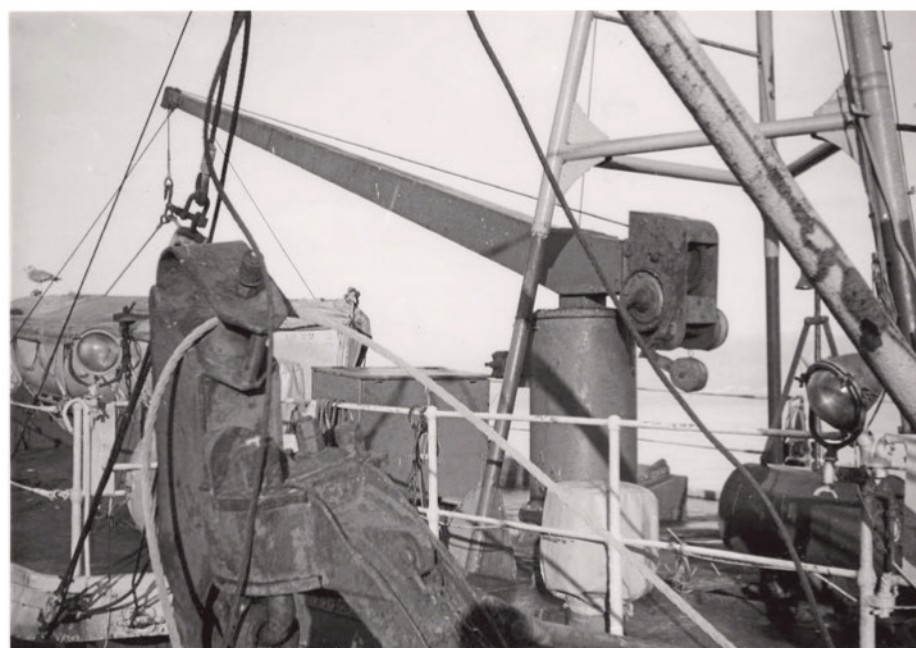
An example of a single arm davit on another vessel.
