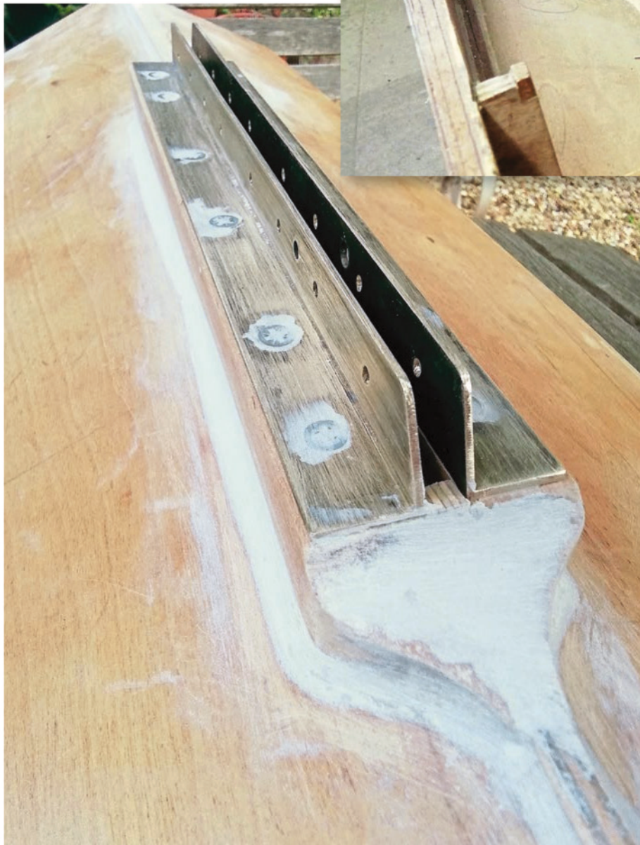
Either side of the keel, a strip of teak was bonded onto the hull, with filler added to blend them in. Two brass angle strips were then screwed onto the wooden strips. The series of holes drilled along the brass would allow adjustment to be made when positioning the keel.
