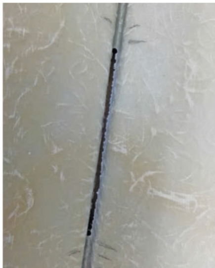
ABOVE LEFT: A slot was cut along the keel line in order to fit a brass keel.
