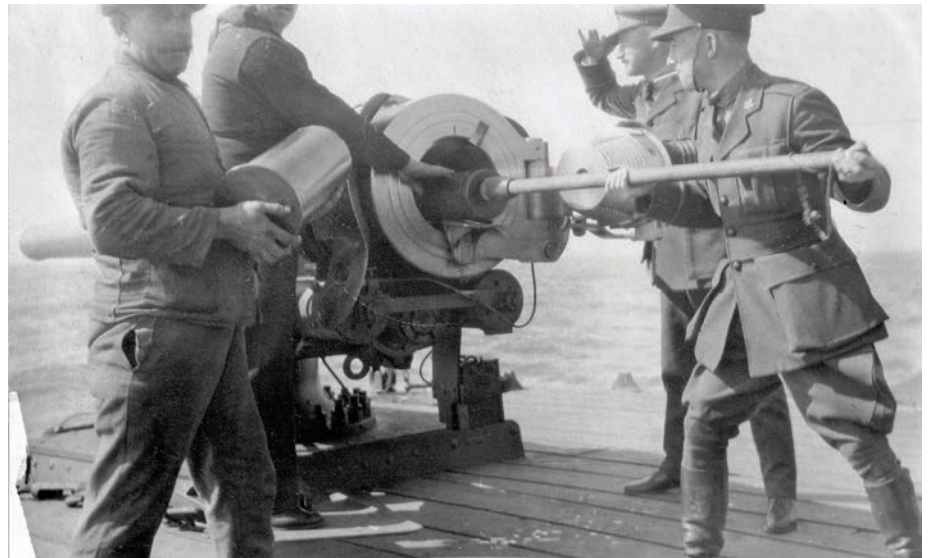
ABOVE: Army officers witnessing the loading and sighting of the 4.7-inch cannon installed on Carpathia to deter the German submarines lurking in the Atlantic.
