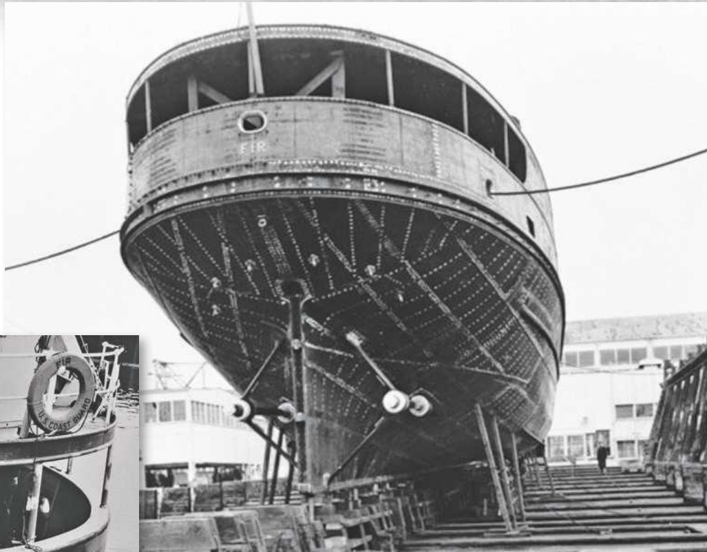
ABOVE: Stern while under construction. Note the especially close spacing of the frames indicated by the pattern of the rivets on the shell plating, and also the propeller extended tubers and supporting brackets. The rubbing strake keep plates have been fitted but not the rubbing stake itself yet.
