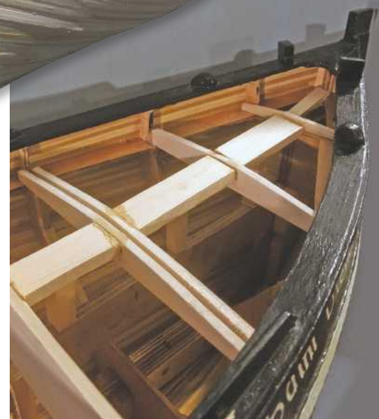
Forward deck beams.
