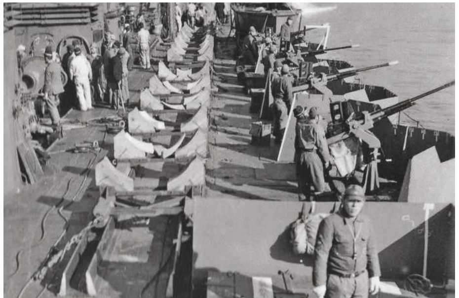
The empty Kaiten deck on board Kitakami , included here to illustrate the robust crutches and handling rails required to launch such a massive craft over her stern.
