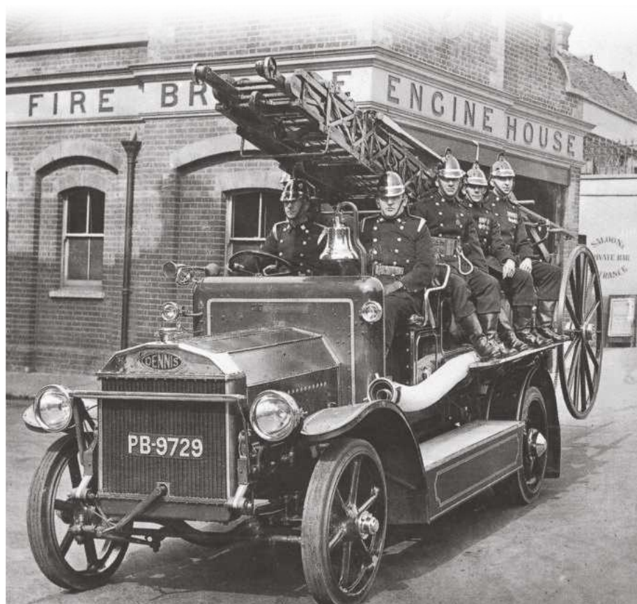
Probably best known for its fire engines, fascinatingly, Dennis Bros did once test the water with a marine fire-fighting installation...
