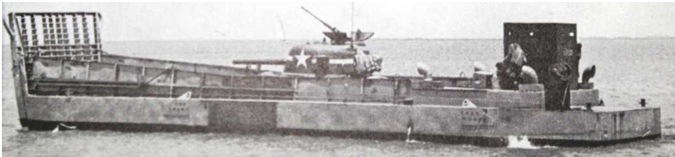
A good example of an LCM(6) showing the 6ft extension to the hull Image courtesy of Allied Landing Craft of World War Two by Arms and Armour Press.
