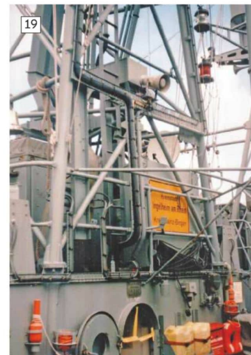
19: The foremast is constructed of a tubular frame with a ladder inside the mast for access to each of the platforms.
