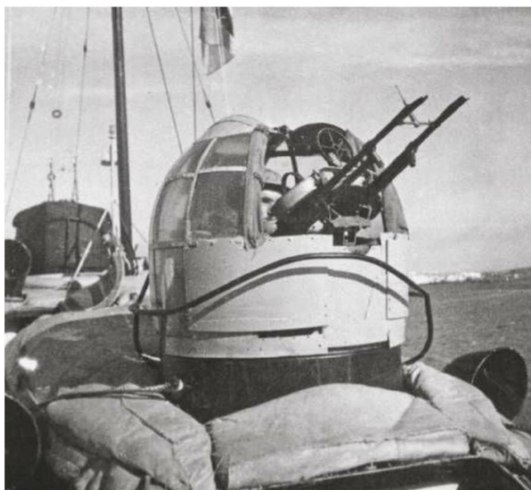
BELOW LEFT: An ASRL turret at the RAF Museum Hendon used for reference. BELOW RIGHT: HSL 128's rear turret showing the suppression rail and the twin machine guns. 'Call-Out' by F R Galea.
