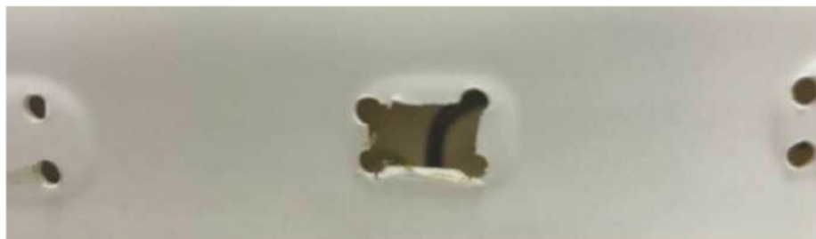
ABOVE: Next in the sequence - joining up the holes.
