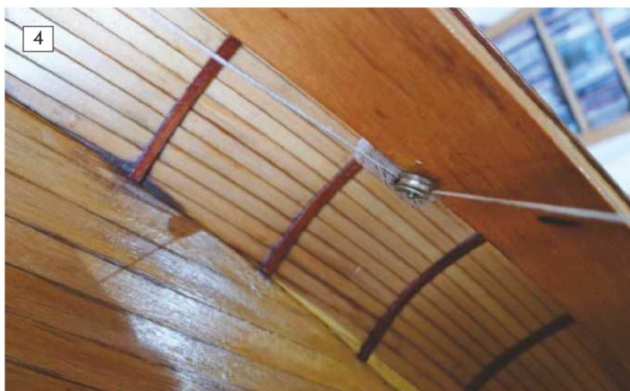
4: The pulley must be in alignment with the cords on either side of it to prevent excessive wear. I mounted mine on a small beech block to give the screws something solid to hold on to.
