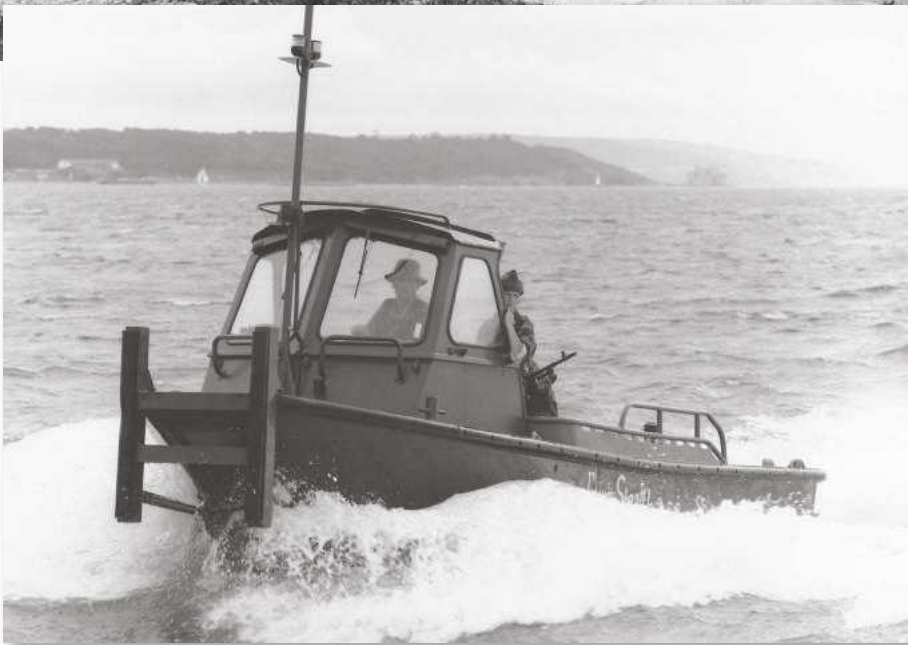
ABOVE: The US Army was impressed by the CSB design and developed a modified version known as the 'Bridge Erection Boat'.
