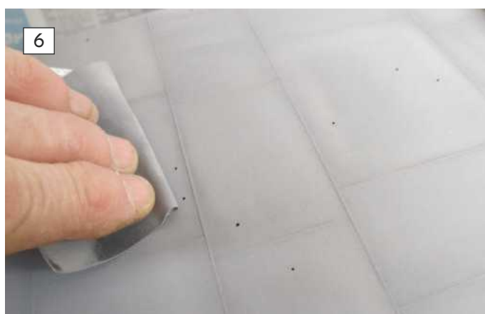
5: Micro Finishing cloth 4000 grade is used to prepare the deck surface for its finishing coat. 6: The primed deck surface is rubbed down with a Micro finishing cloth.
