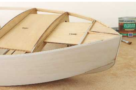
ABOVE: As you can just about see, the deck takes a slight dip at the front; another area for careful profiling.
