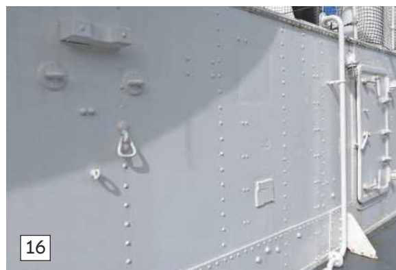
15 & 16. Note the detail on the bulkhead beneath the boat stowage platform. The purpose of the brackets and lugs is not known.
