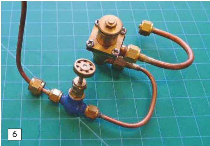
ABOVE LEFT: Complex pipe runs can be separated by the fittings to make the individual pipes much easier to make. This assembly is simply a collection of straightforward bends, the most complex being an S-bend.
