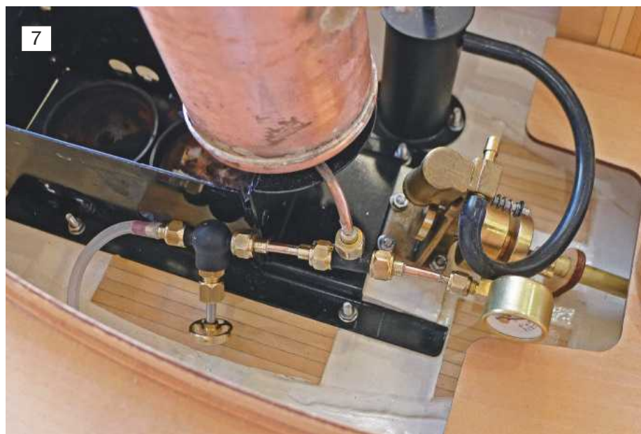
Photo 7. With a folding boiler, the operation of lifting it up cannot be interfered with and so the manifold had to clear all the internal components when in that lifted position.
