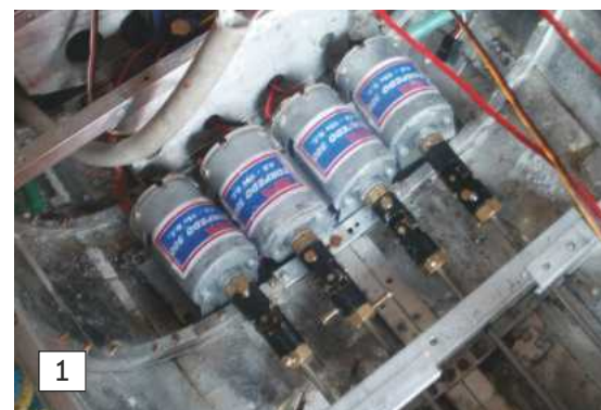
Photo 1. A rather sad looking temporary electric motor installation - the mountings are just held in place on a bed of silicone bath sealant to the hull's internal bottom. Not perhaps what you would expect of 'proper' model engineering, but quite practical in the circumstances.
