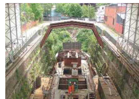
Above: Medway Queen hull is well on its way to completion, May 2011. (Photo courtesy of David Abels)
