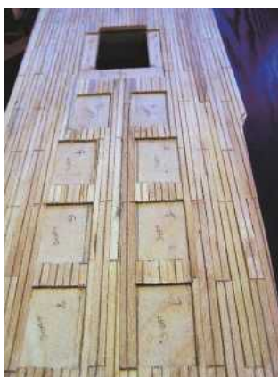
Above: The planked promenade deck with cut-outs for superstructure components
