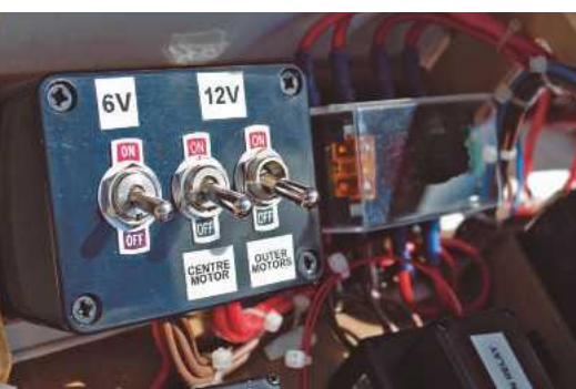
Above: Ray has put all the electrics into dedicated boxes for ease of maintenance and knowing 'what's what'.
