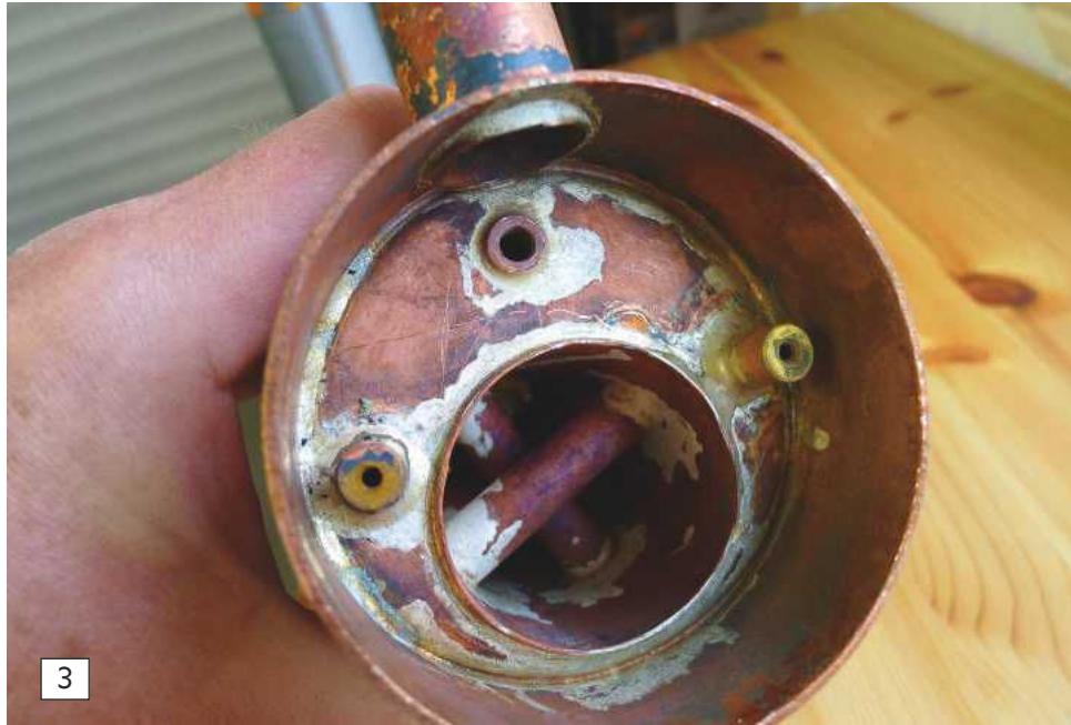
Photo 3. When the boiler was received back from repair, it was complete with two new tapped bushes perfectly soldered in the end cover of the boiler, ready to take the new screws.
