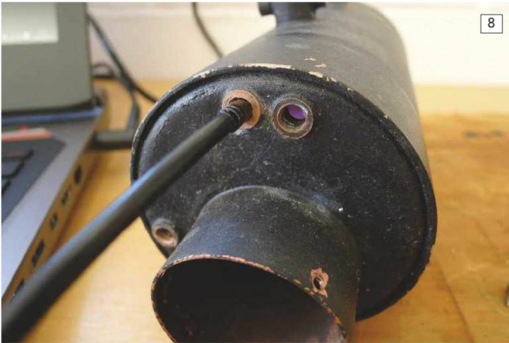
Photo 8. The head of the Borescope is just 5.5 mm making it suitable to pass through quite small boiler mounting bushes. The device increases the scope of what can be viewed inside and gives a good idea of the boiler's internal condition.
