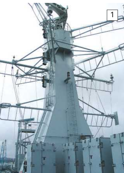
Photo 2. The foremast arrangements showing the air search radar and UHF arrays ringed in red.
