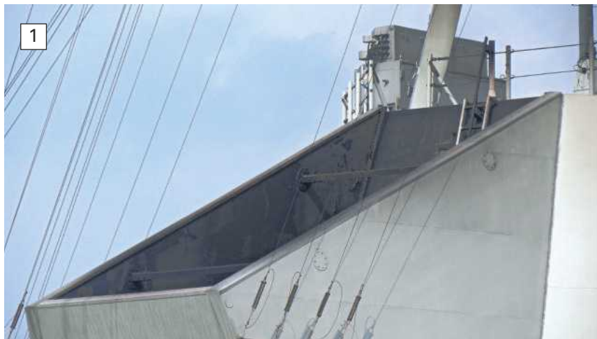
Photo 1. Looking towards the top of the forward exhaust stack.
