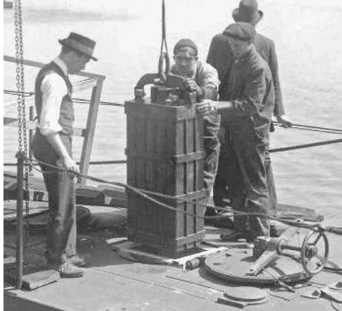
LEFT: Installing a battery cell in an American L class submarine, 1916. Note the protective gloves for the workmen, but not much else! (US Navy official photo)
