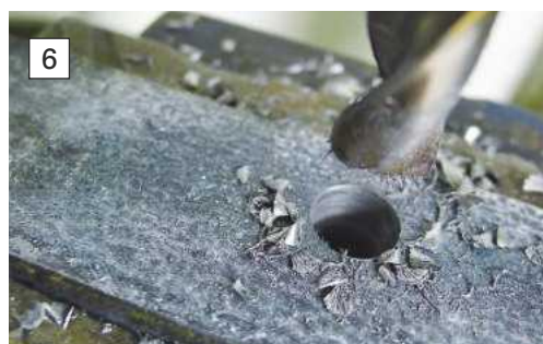
PHOTO 6. When you finally back-off the drill bit, you should be left with a neatly cut hole that is uniform in diameter and in just the right location. Heat generation should have been minimal, but the drill bit and the job could still be quite warm for some time afterwards.
