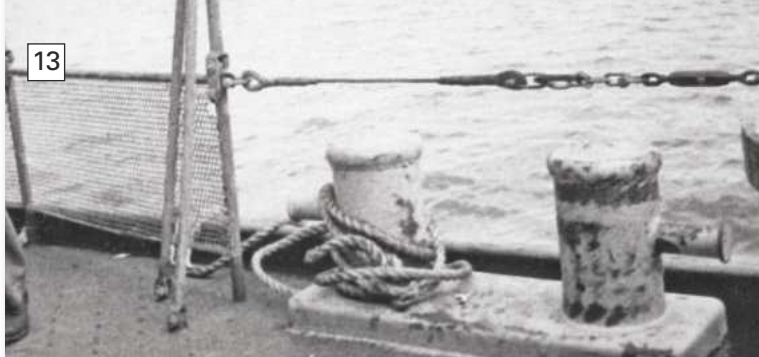
PHOTO 13. Bollard and stanchions as fitted to T35.
