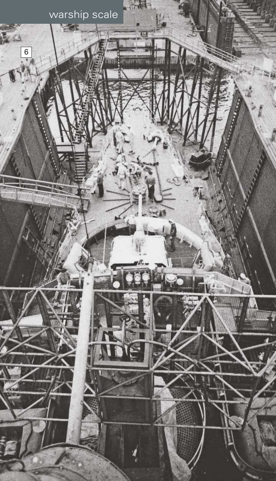
PHOTO 6. Looking down on to the radar scanner 'mattress', the open bridge and the forecastle.
