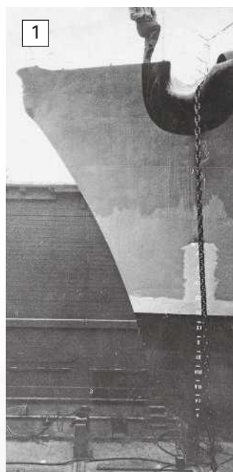
PHOTO 1. The bow and deck edge anchor arrangement.
