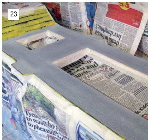
Photo 23. Masking of the upper deck, now with conventional tape and newspaper.
