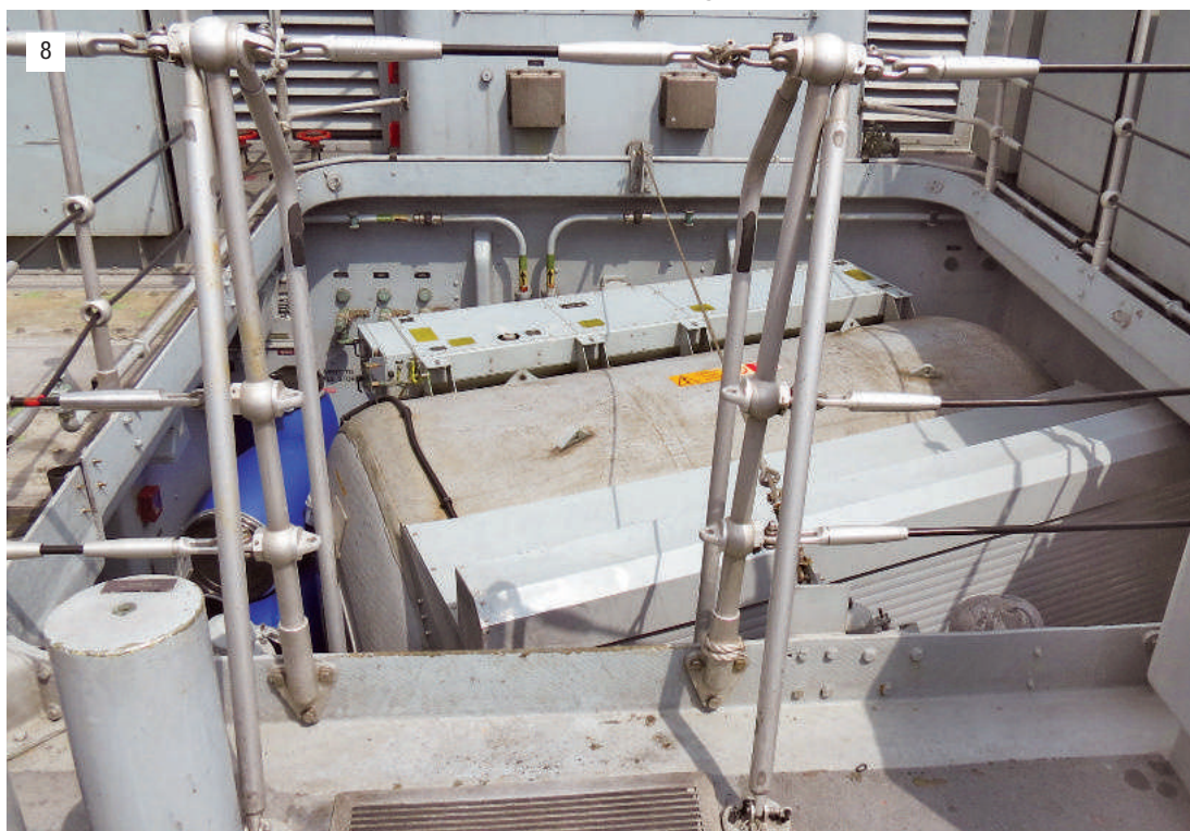
Photo 8. The open well on 01 deck is above the decompression chamber.
