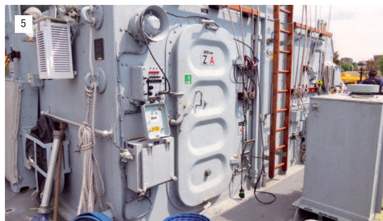
Photo 5. On 01 deck, the housing supporting the mast has a huge number of surface fittings.
