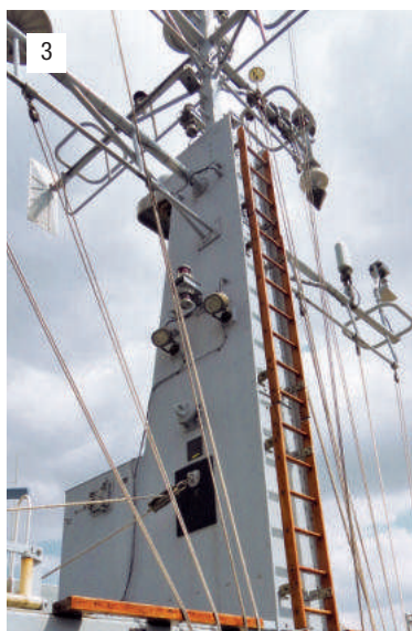
Photo 3. A wood ladder is used to gain access to various sections of the mast and its fittings.
