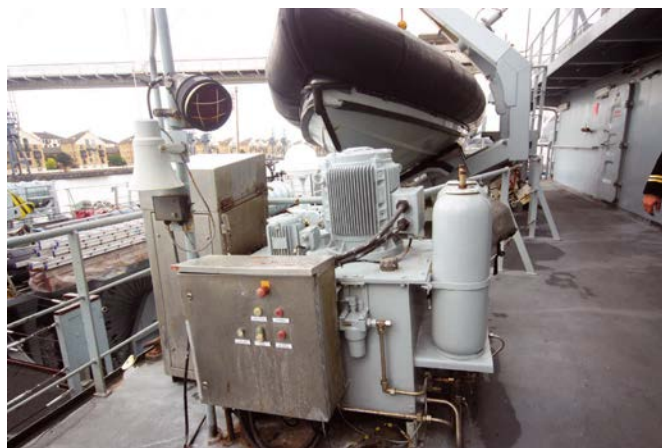
Starboard side amidships looking aft – note one of two rigid raider fast intercept craft on its davits used to board and inspect fishing boats
