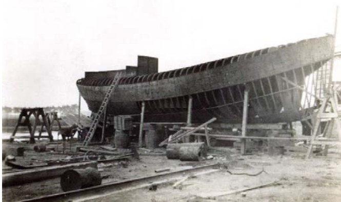
Starboard view during construction
