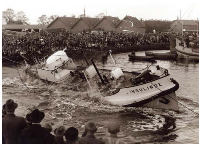
105 seconds after deliberately capsizing 'Insulinde' she was up and afloat again. Snapshot taken in Delfzijl on the 27th April 1927
