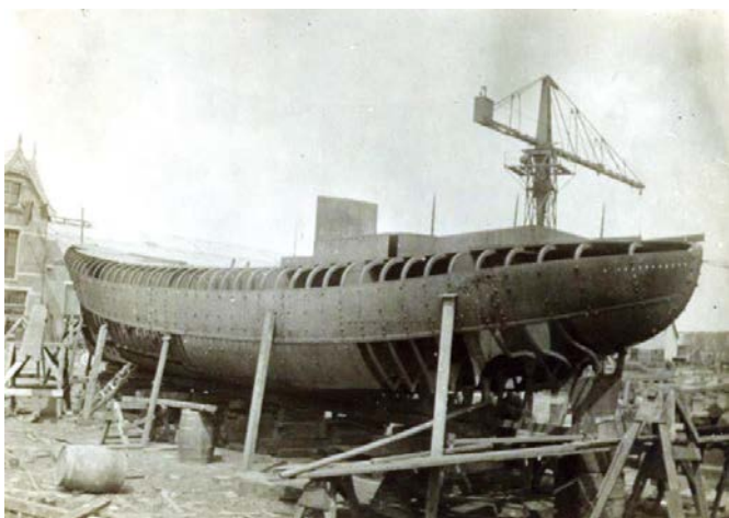
The tunnelled props in a portside view
