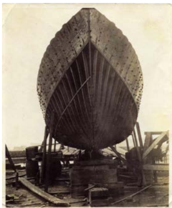
Front view of 'Insulinde' during construction at Gebroeders Niestern yards at Delfzijl
