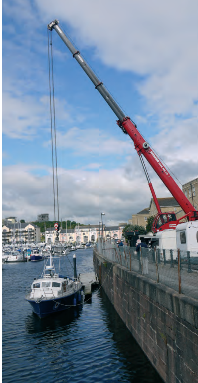
Made ready for the lift
