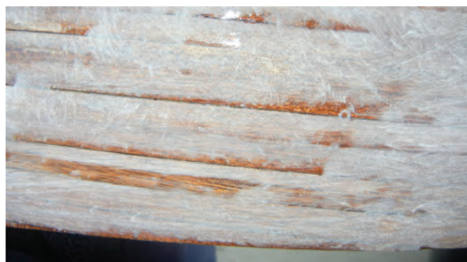
ABOVE & BELOW: Applying and sanding mahogany planking veneer
