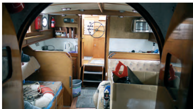
The saloon is rather untidy due to the work taking place
