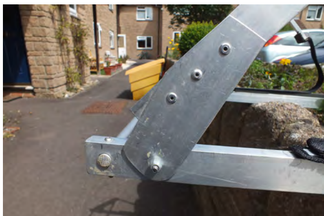
Bottom aluminium tube blocked (tube can be extended to fit wheels)
