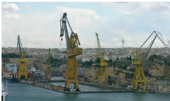
The huge China drydock photographed in 2010; measuring 1170 by 195 ft with a handling capacity of 300,000 DWT
