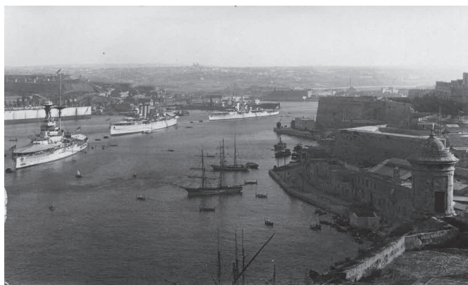
Looking down from the Upper Barrakka Gardens with AFD VIII visible on the far left
