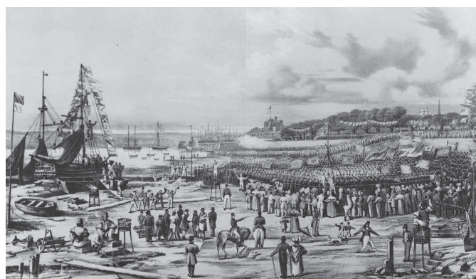
Laying of the foundation stone 1836 (BTC/ABP)
