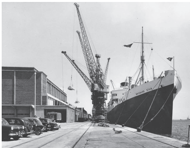
Brisbane Star at the new Cold Store on berth 108 (BTC/ABP)
