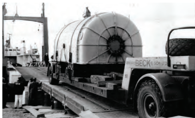
Here we see the winch cable attached to the rear of the transporter truck (photo courtesy Edward Beck)
