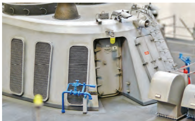
Ventilation, steps, doorway and communication detail around the funnel room enclosure
