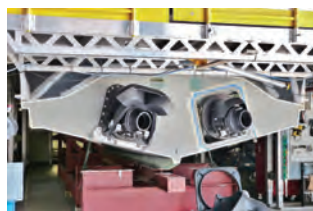
Below the upper floor level engineers can work on the external aspects of fitting the Hamilton HJ364 water-jet units, each capable of absorbing 770 hp of pressure
