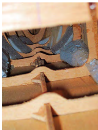
View of foam infill inside hull
