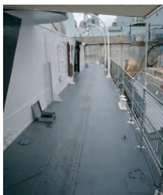
Deck on port side showing deck plates riveted
