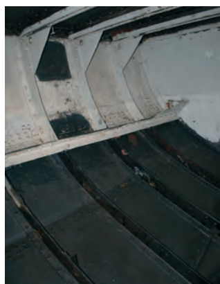
Showing the rivet construction
