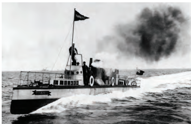
The Turbinia at speed
