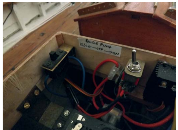
Three position switch for either pumping out when alongside, electronically via a spare radio channel while at sea or off
