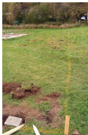
The boundary for the new pond marked out
