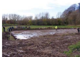
Rather muddy excavations complete!
