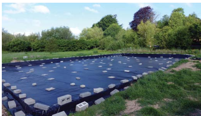
Liner now held in position waiting for the water
