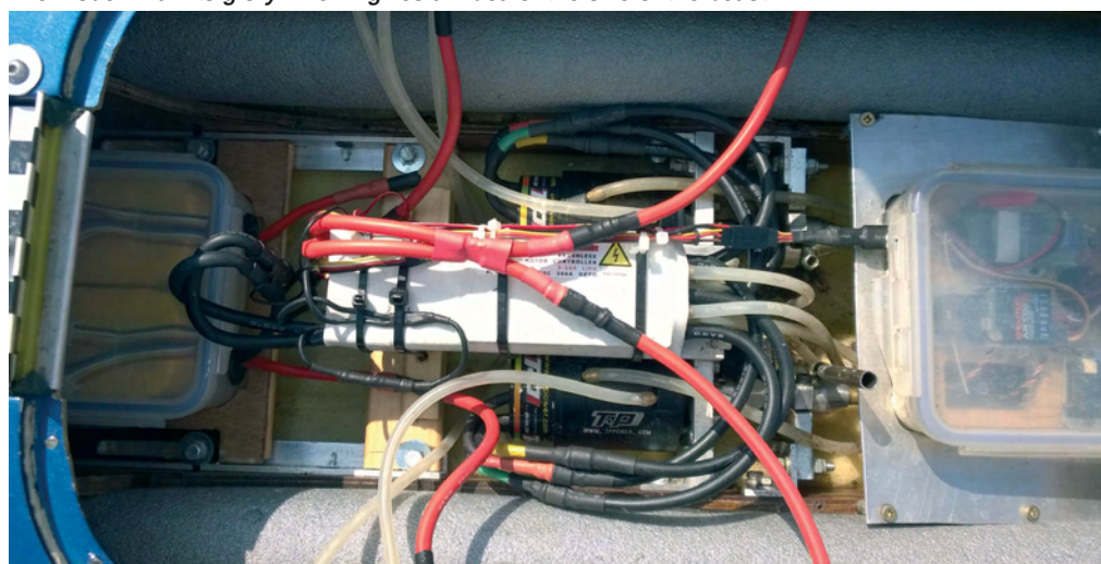
General view of the interior. Lots of wiring. Note waterproof boxes for radio and cells
