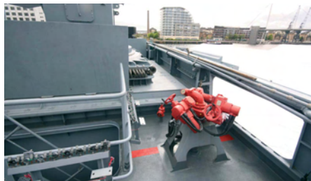
Fire hydrant under rear RAM launcher
