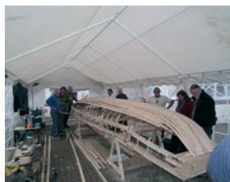
Longitudinal strips of wood stapled onto the ribs
