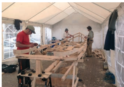
Work starts on the gunnels in the temporary marquee
