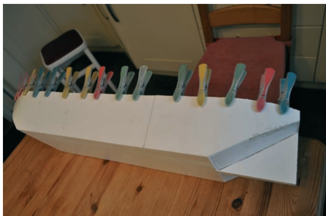
Plenty of pegs and clamps required to hold the cladding in place while the adhesive sets
