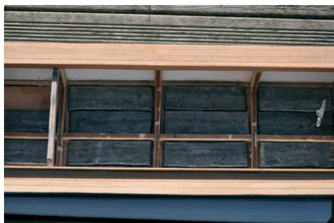
Deck now planked and lead sheet ballast installed
