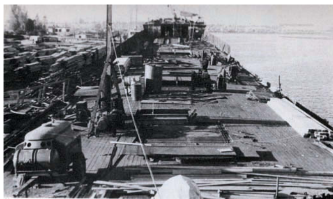
Now named Tango, this is Hans in September 1941, being converted back from a gambling hulk in San Francisco. Her midships Liverpool house has gone, and her bulwarks are being re-built
