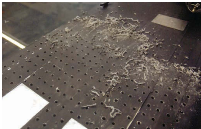
Aft 'metal' deck drilling
